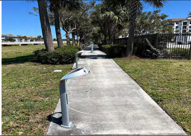
Photo 37: Greenway-West End Looking east
