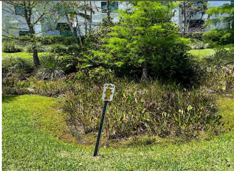
Photo 5: Steep bank with sign-outfall needs excavation.
