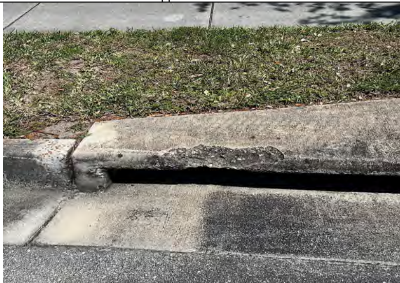
Photo 18: Chipped inlet top should be patched on RCBN.
