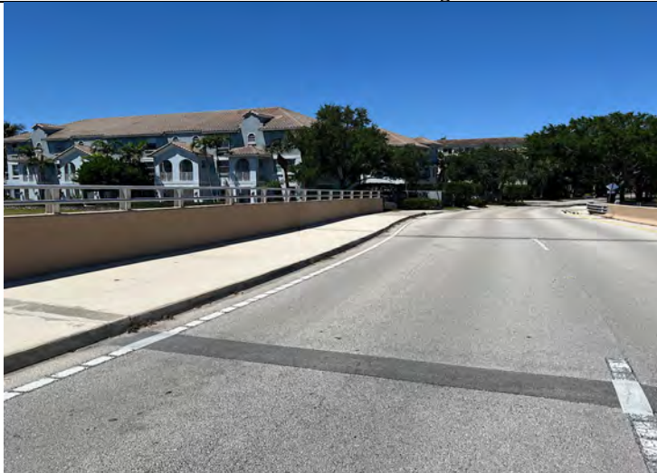
Photo 35: RCBS at Bridge
