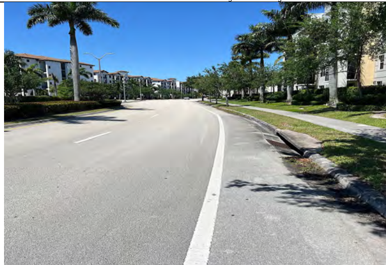
Photo 26: Dirt in Gutter RCBN North of Dog Park
