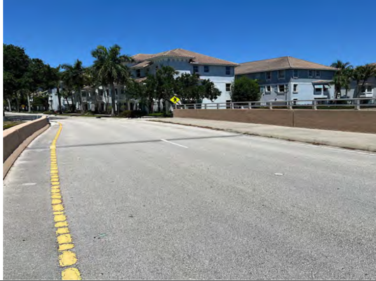
Photo 34:RCBN at Bridge
