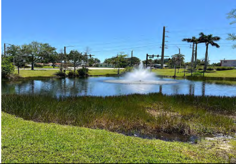
Photo 1: Aerator working well.
