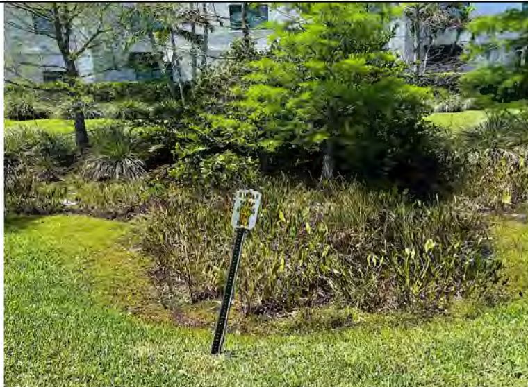
Photo 5: Steep bank with sign-outfall needs excavation.
