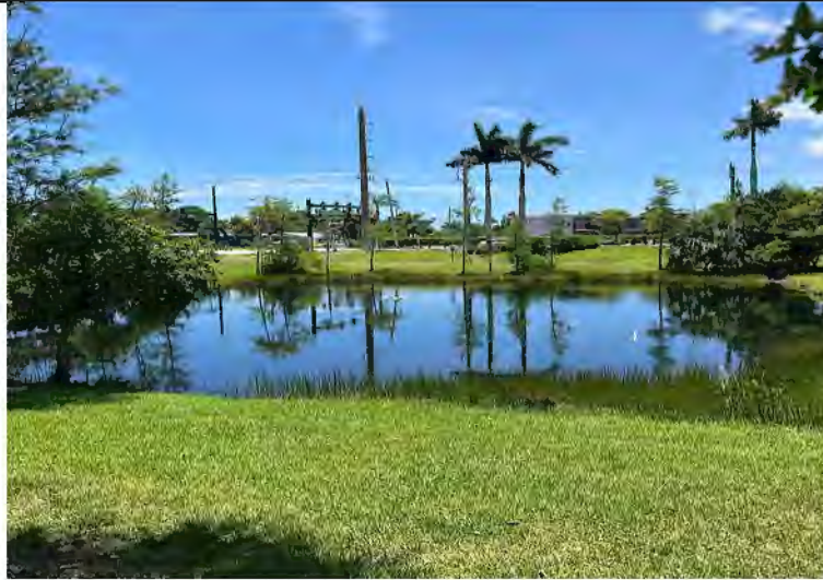
Photo 1: Aerator not working.
