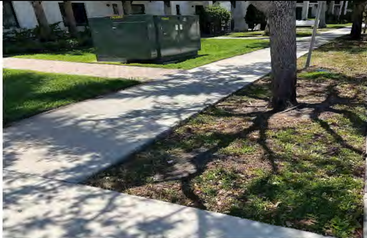
Photo 22: Drop off by walk presents fall/trip hazardt RCBS between bridge & Audace Ave
