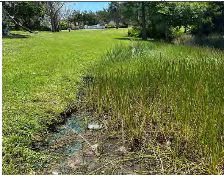
Photo 2: Steep bank drop-off.
